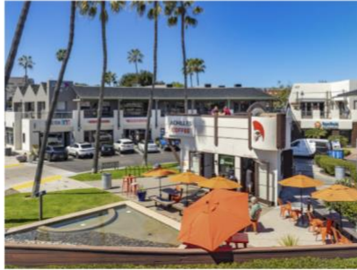
Beachwalk Shopping Center in Solana Beach, Calif., offers 55,580 square feet of retail, restaurant, medical and creative office space.
