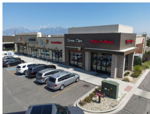
Trail Crossing Shopping Center in South Jordan, Utah, offers 38,397 square feet of retail space.
